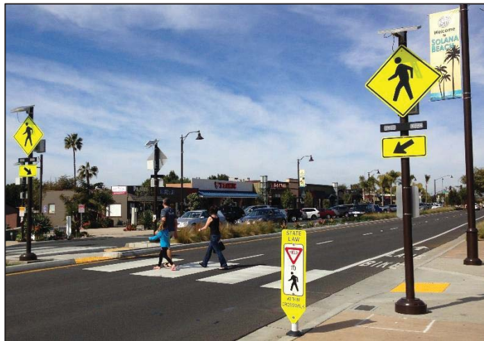
Four (4) additional pedestrian crossings were installed as part of the Highway 101 Revitalization Project completed in September 2013.
