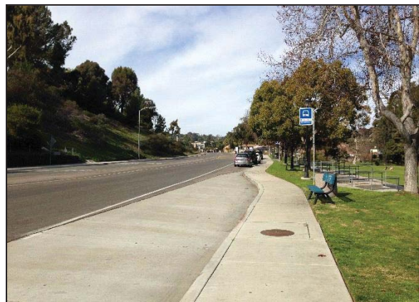
La Colonia Park is one of Solana Beach’s recreational resources currently inaccessible by existing bicycle facility.
