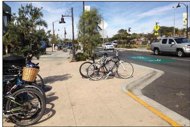
Bike racks, a green-backed sharrow, pedestrian scale lighting, high visibility pedestrian signs, and a mid-block crossing are features all present in this image of Highway 101.
