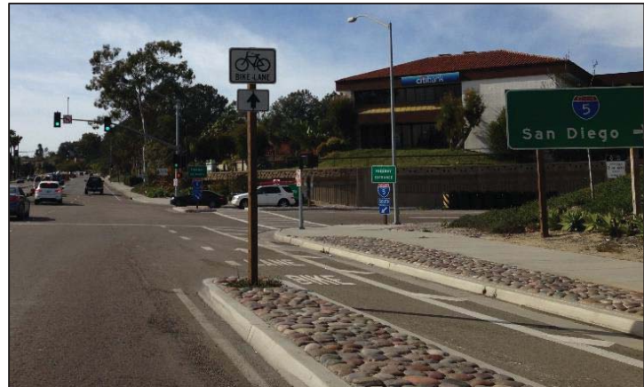
Bicycle and pedestrian collisions were recorded on Lomas Santa Fe Drive near Interstate 5.
